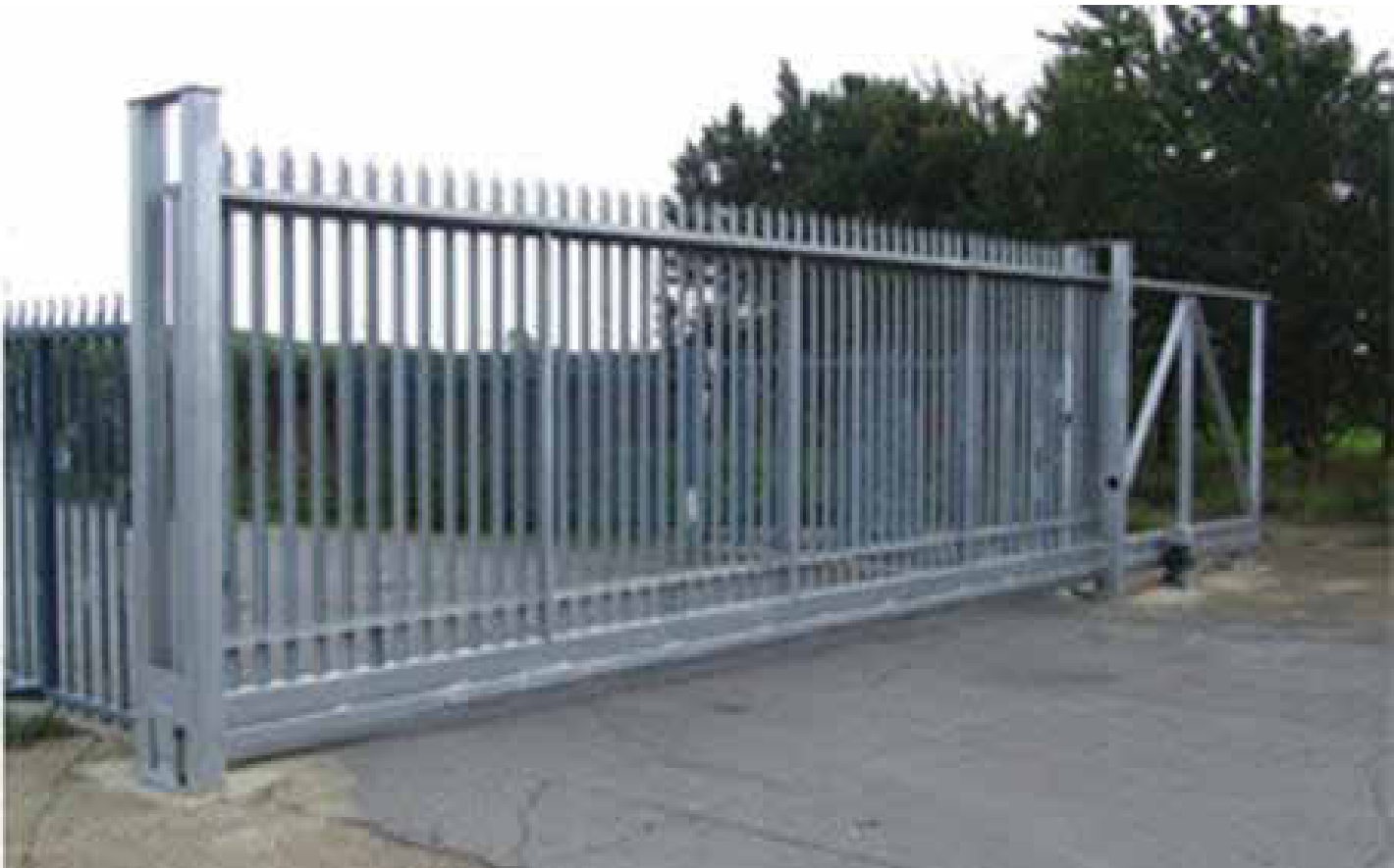
Proposed Yard sliding gate design. Approx 8m wide x 2.4m high (2.6m total height) to match proposed fencing.
